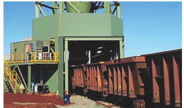
Loading ,Unloading & Train Station
