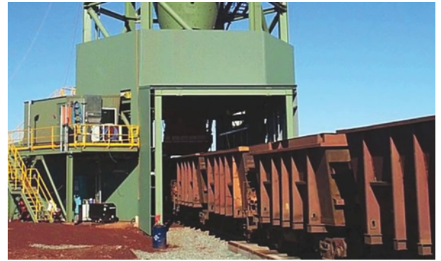
Loading ,Unloading & Train Station
