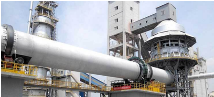
Cement Rotary Kiln
